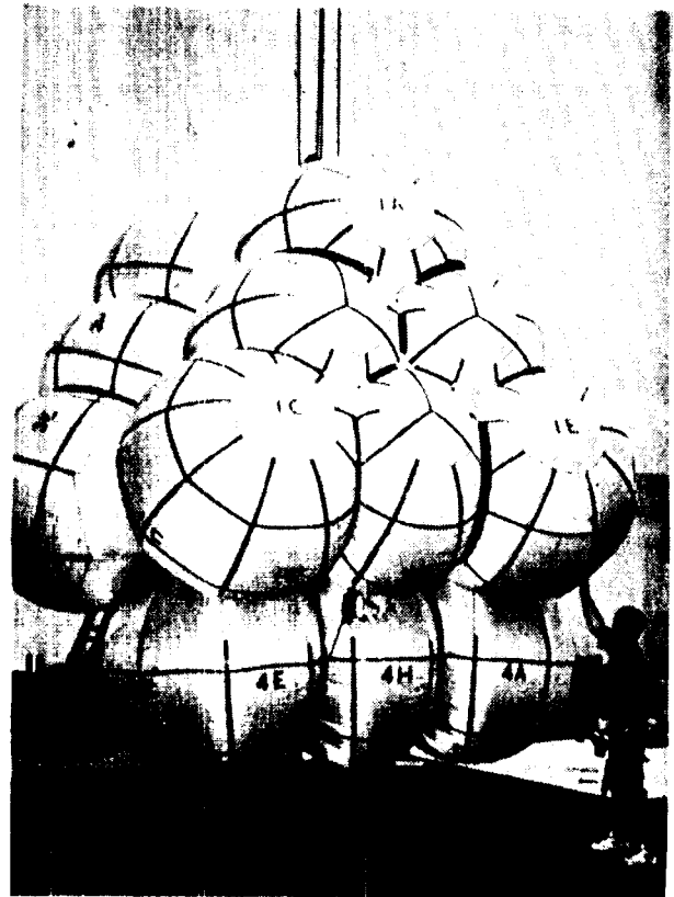
Fig 4: Flight Prototype Airbag/Lander System
