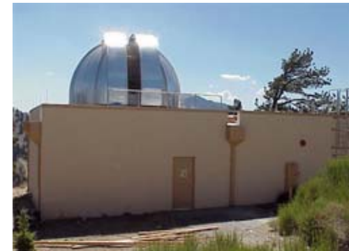
Optical Communication Test Laboratory (OCTL)
