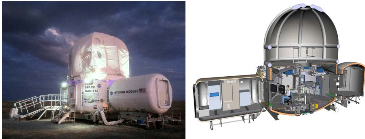
Figure 1: Habitat Demonstration Unit, 2011 D-RATS configuration with U. Wisconsin X-Loft (left), section (right)
