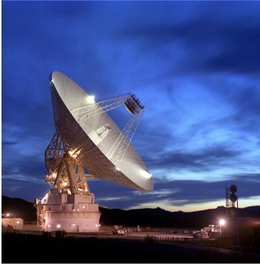
**Figure 1: A 70-meter antenna in the NASA's Deep Space Network**
